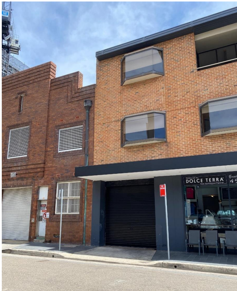
Photograph of loading dock and waste room – located off Short Street
