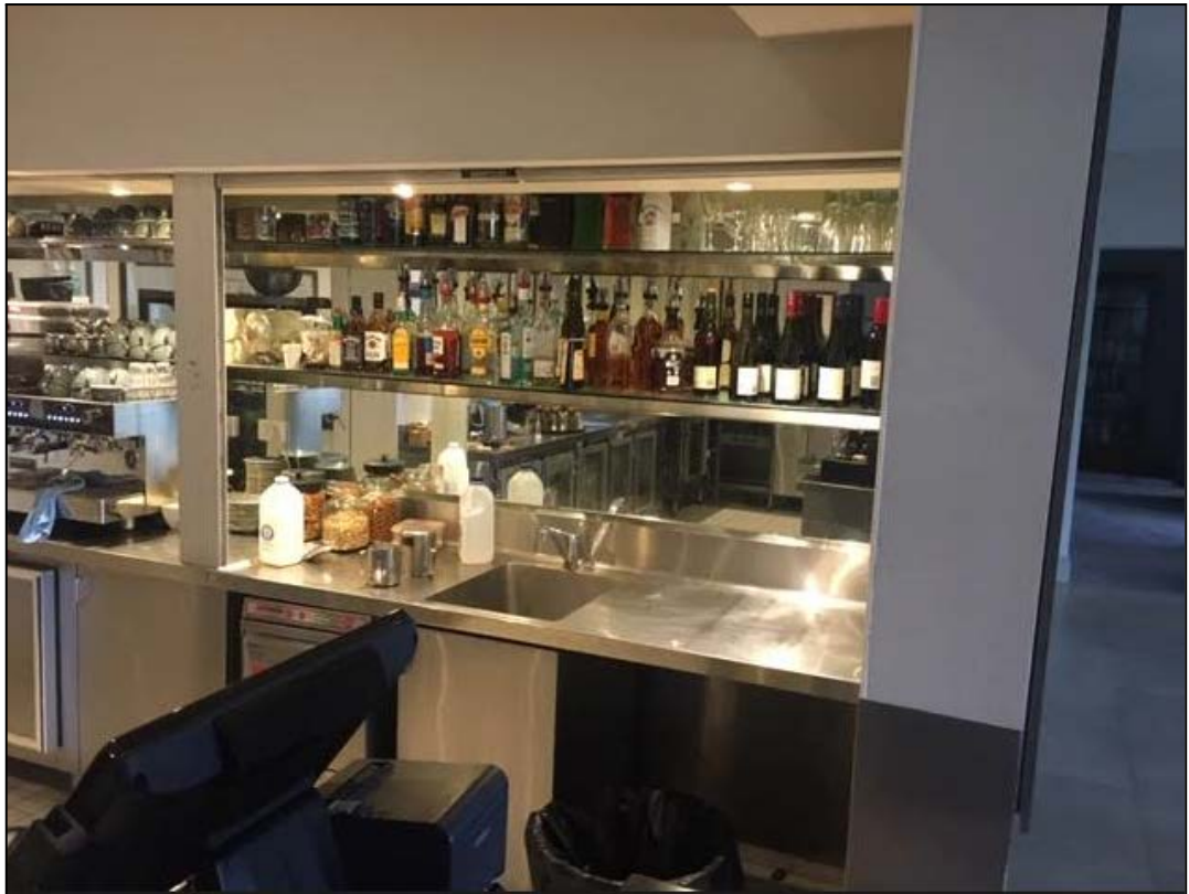
Figure 5: This section of bar including the wall will be removed. The wall is not structural.
