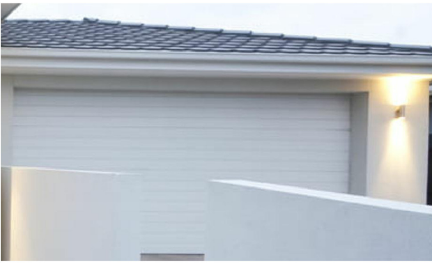
GARAGE DOOR: COLORBOND HORIZONTAL PATTERN WHITE FINISH
