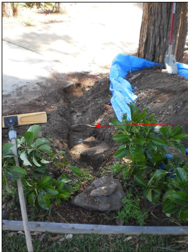
Photo B: Trench facing north east.
