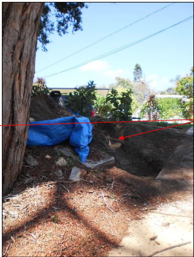
Photo C: Trench facing west.
