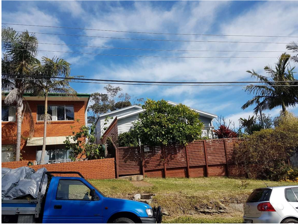
Figure 1: View of the site from Dowling Street.
