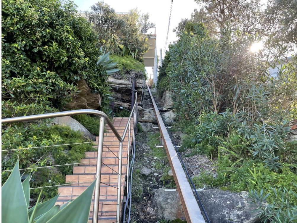
Fig 10: View of the existing inclinator (which is to be retained and extended to the new entry foyer at road level) looking upslope to the west
