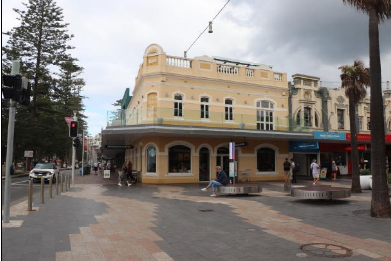
Figure 5: Nos. 110-112 The Corso to the north of the site, a two-storey Victorian period former hotel, now used as shops.
