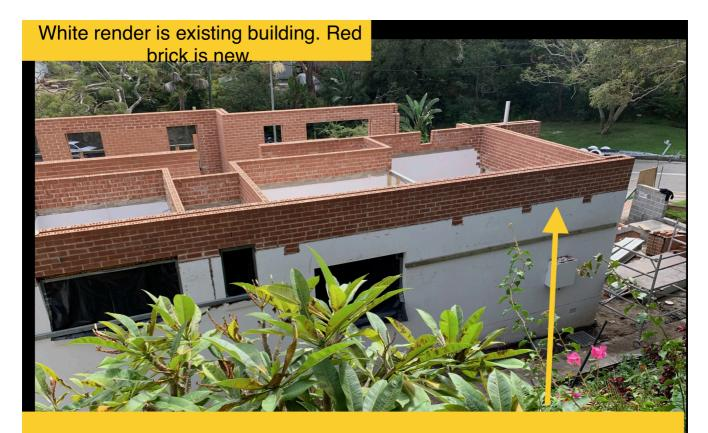
8 courses of brick has added an unauthorised 688mm in height to the existing external Eastern wall (76mm brick +10mm of mortar =86mm x 8 brick courses high). The Western walls are newly built atop new foundations and a new slab. This level (first floor) will have an additional 400mm slab on top of the 8 brick courses. This equates to an unapproved breach of 1088mm. The entire Western boundary wall has been newly constructed over a meter higher than what was previously existing.
