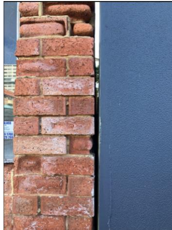
Figure 6: Separate walls between adjacent gym and commercial buildings
