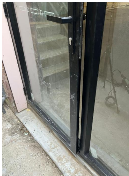
Figure 32: Recommended door to be treated with acoustic seals (facing Parkview)
