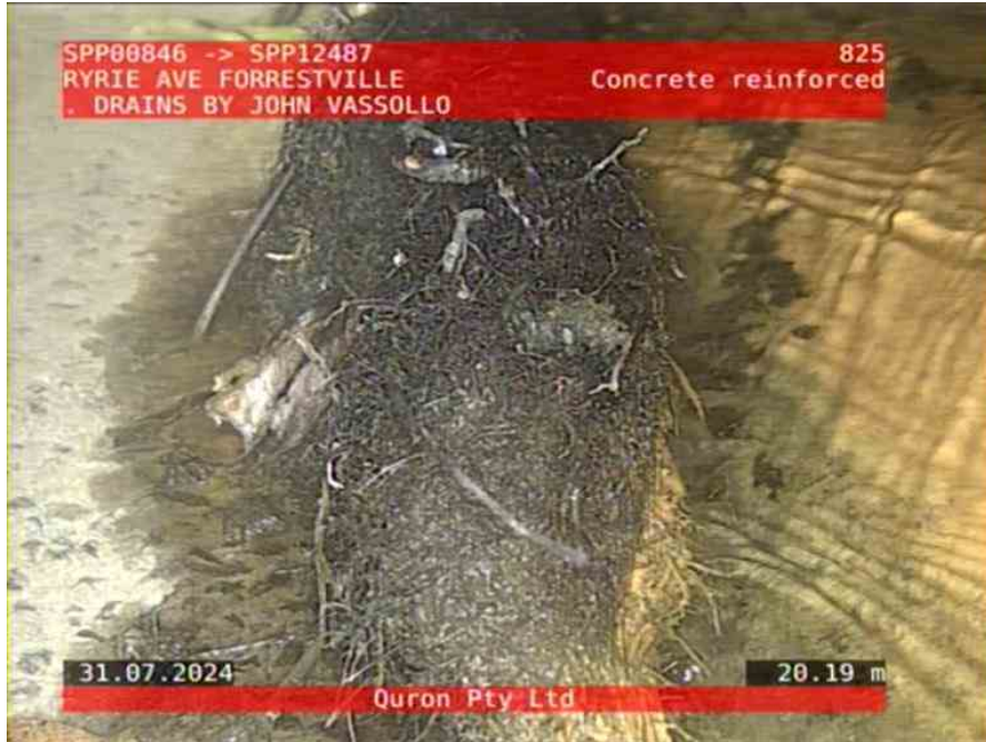
SPI13382_7292854f-d61e-4683-b0d1-0b4fb2d17d08_20240731_112515_449.jpg, 00:06:35, 20.19 A mass of mostly fine roots, which has developed into an interwoven clump, at joint, Obstruction: 5-20% at 7 o'clock
