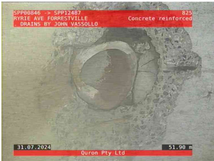
SPI13382_4a330966-c5b3-497e-8065-c1db63970d04_20240731_113308_437.jpg, 00:12:53, 51.90 Connection, poor workmanship, connection appears to be open, height: 100mm at 10 o'clock
