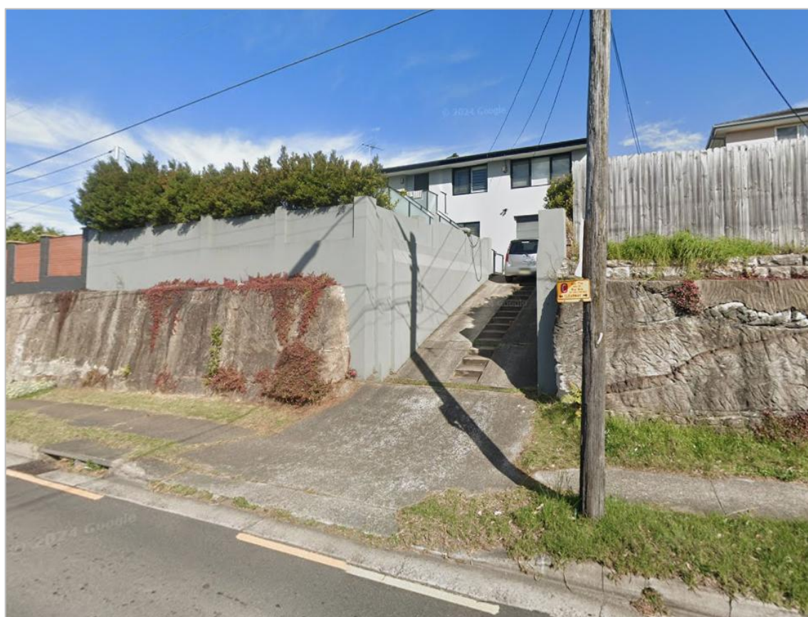
Figure 2: Existing Dwelling and Driveway
