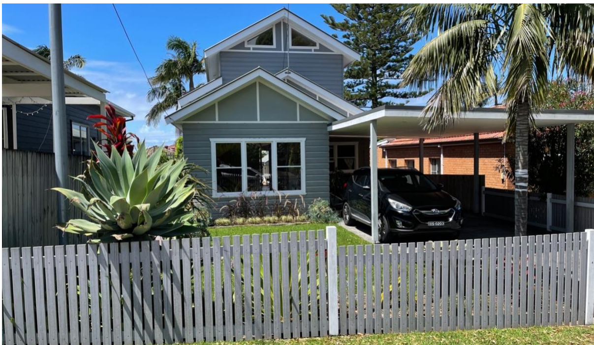
Figure 7 – Neighbouring site at 7 Aubreen Street (Dragonfly Architects, 2021)
