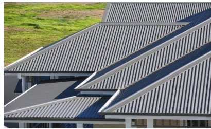
COLOURBOND METAL ROOF SHEETING POWDERCOAT FINISH 'IRONSTONE' OR SIMILAR WHERE MARKED ON ELEVATION.
