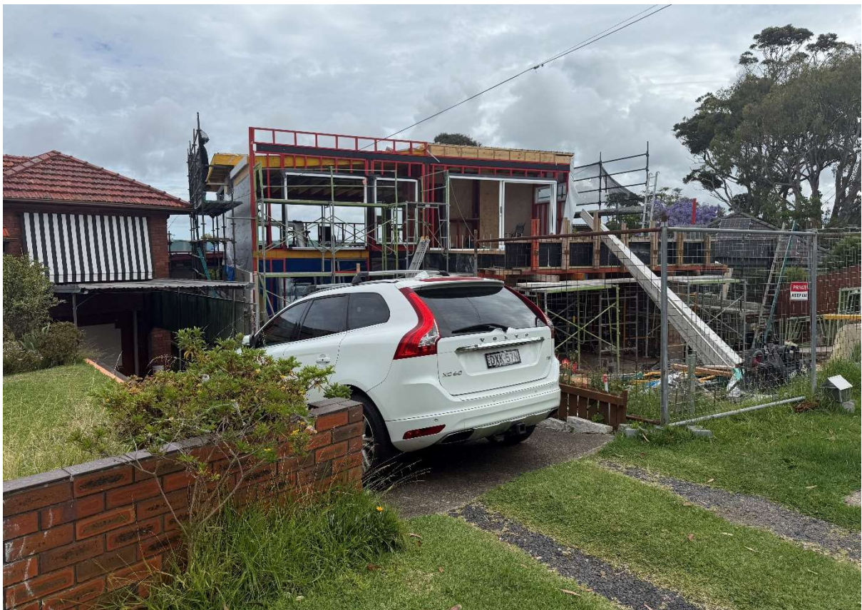
Figure 4 – The existing dwelling (left) and the neighbouring dwelling under construction (right) Source: NBP
