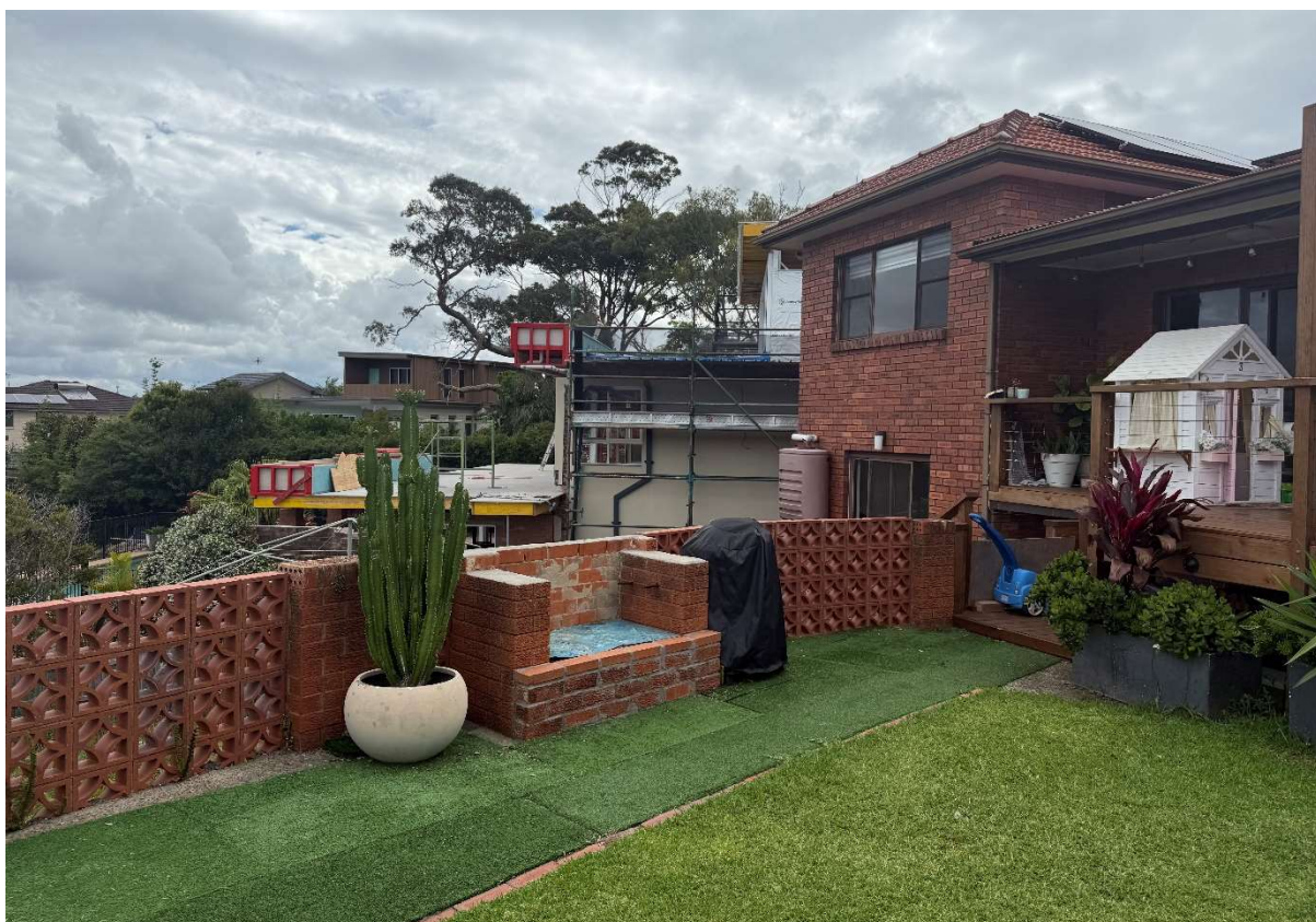
Figure 5 – The rear of the existing dwelling (right) and the neighbouring dwelling under construction (centre) Source: NBP
