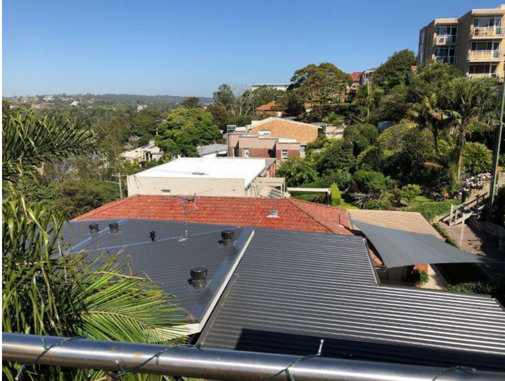
Figure 11 – existing view to the west from existing front roof-top terrace
