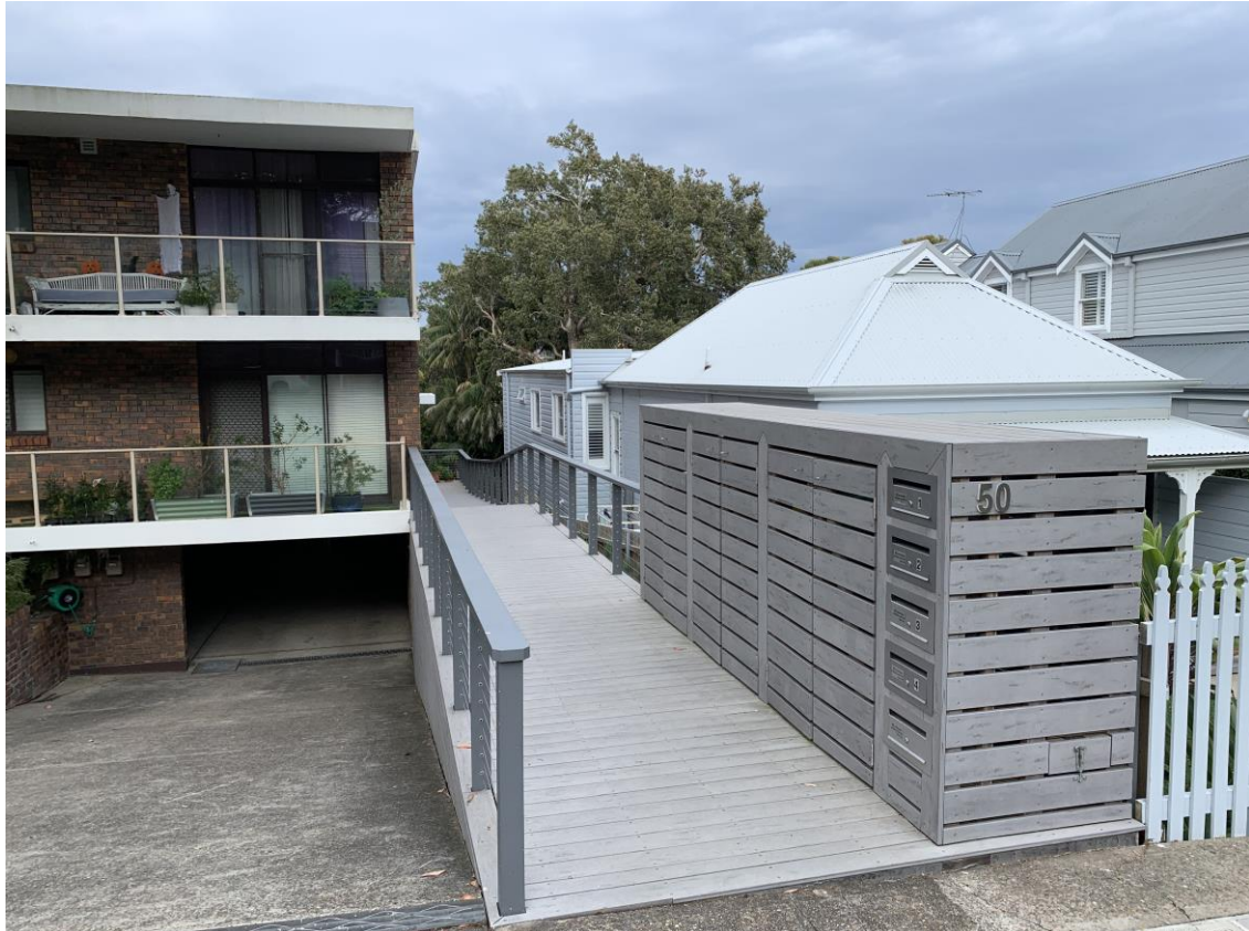
Fig 5: View of the existing boundary structures with the neighbouring site at 18A Marshall Street and adjoining the proposed works within the subject site
