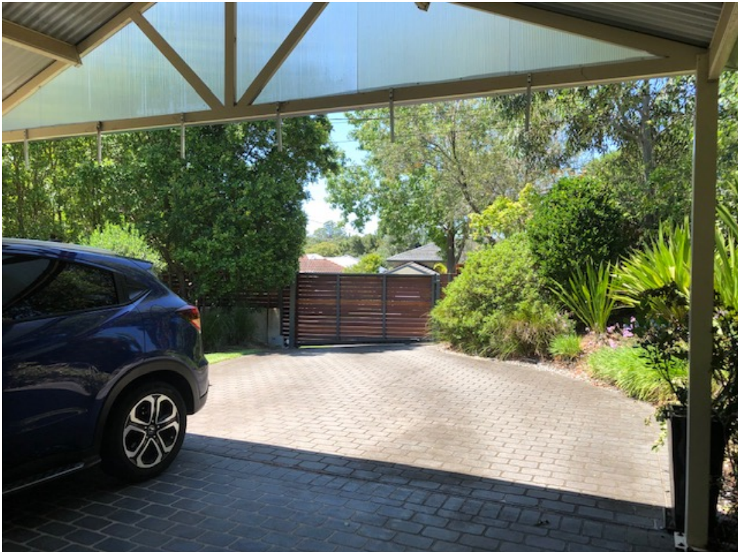
View of existing carport & driveway towards Larne Place
