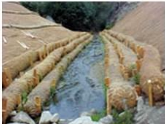
Photo 19 – Creek embankment stabilisation example.
