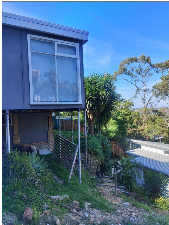
Figure 6: View towards south east from rear of dwelling (source: SKY Town Planning)
