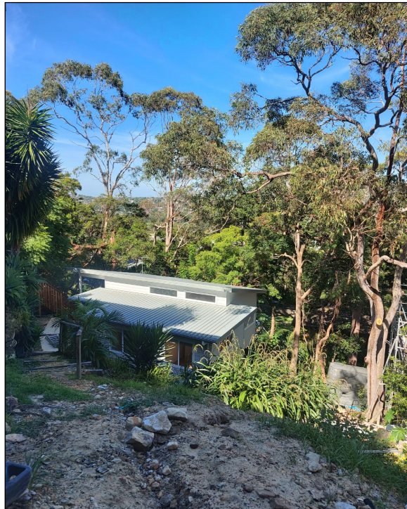
Figure 3: Rear view to the existing secondary dwelling (source: SKY Town Planning)
