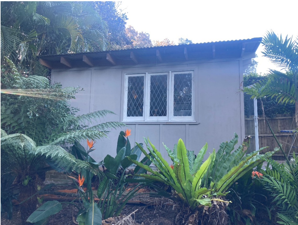
PHOTO 2 – EXISTING CABIN 1 SOUTH WALL
