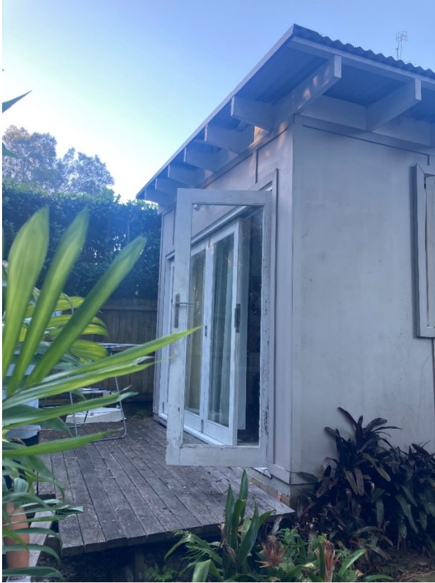
PHOTO 1 – EXISTING CABIN 2 WEST WALL
