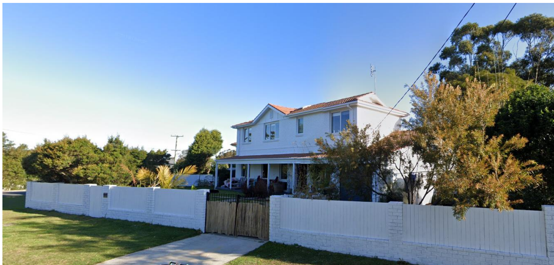
Figure 6: No. 32 Monserra Road, viewed from Cootamundra Drive
