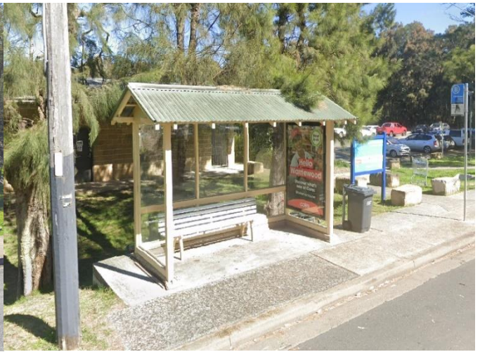
Figure 5 Existing B4 Bus Stop and Shelter on Jacksons Road
