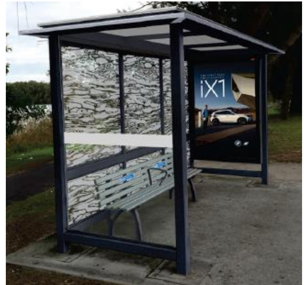
Figure 11 Typical Static/Static shelter installation
