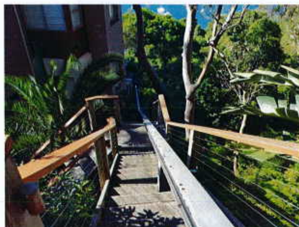
Inclinor & Stair Access, looking N
