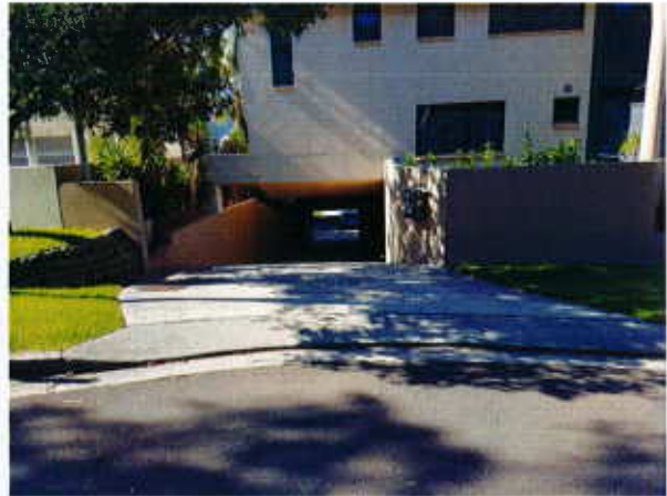
Existing driveway / vehicle access
