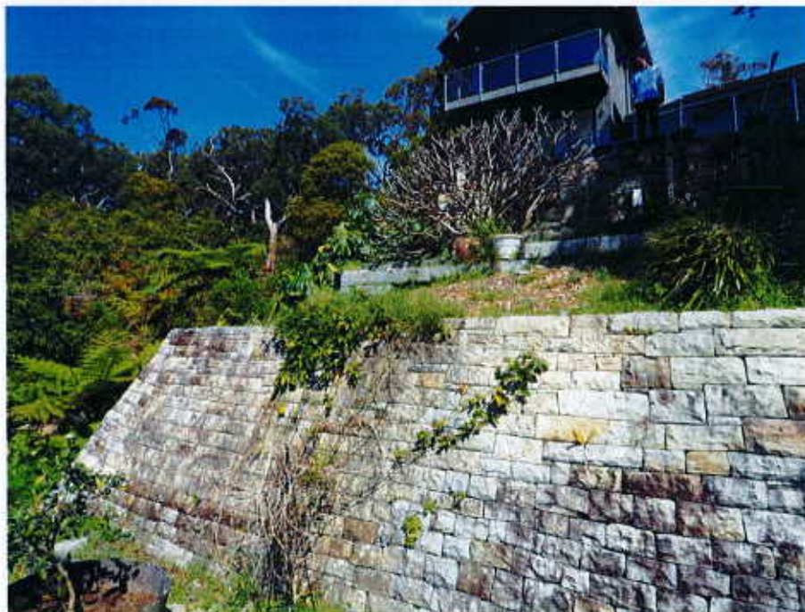
Rear Private Open Space & Dwelling Elevation (Looking Southwest) Note sandstone wall in foreground to be retained.
