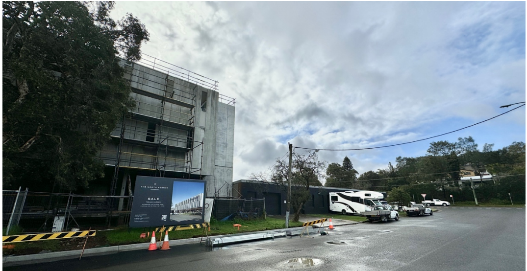
Tengah Cr looking North West
