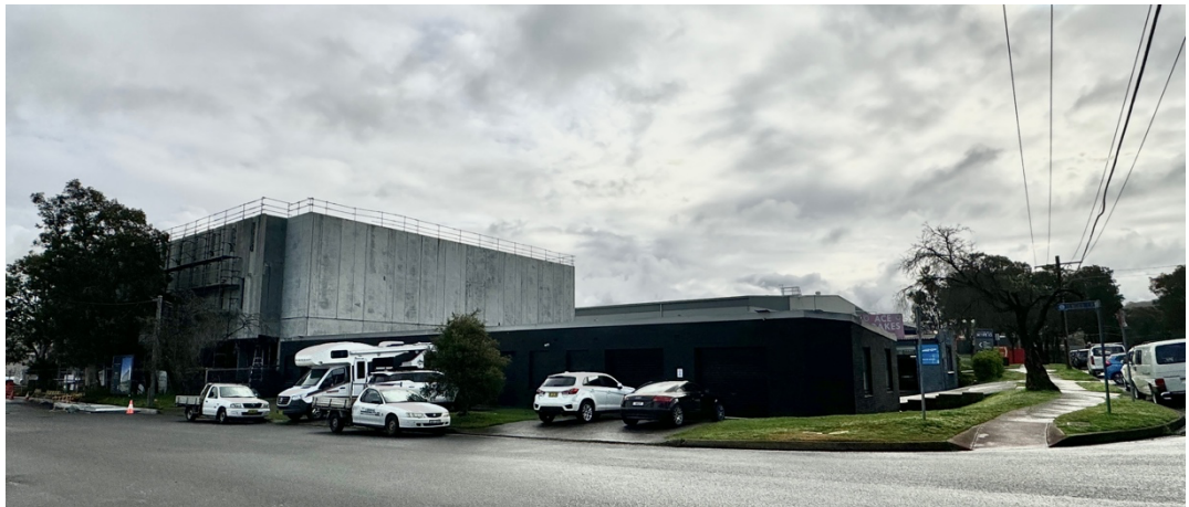
Tengah Cr looking South West
