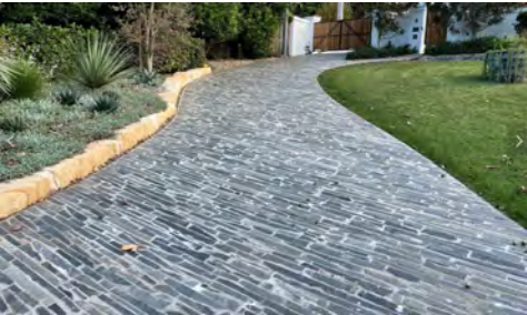
ST-01 STONE TILE ON DRIVEWAY,FOOTPATHAND EXTERIOR STAIRS. COLOUR TO BE CONFIRMED BY CLIENT WHERE MARKED ON ELEVATION/PLANS.
