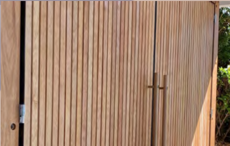
TB-01 TIMBER VERTICAL BATTENS TO BE INSTALED ON DOORS AND FACADE. COLOUR TO BE CONFIRMED BY CLIENT.
