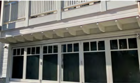
WI-01 TIMBER FRAME BIFOLD WINDOWS AND DOORS. COLOUR TO BE MATCHED EXISTING. WHERE MARKED ON ELEVATION/PLANS.
