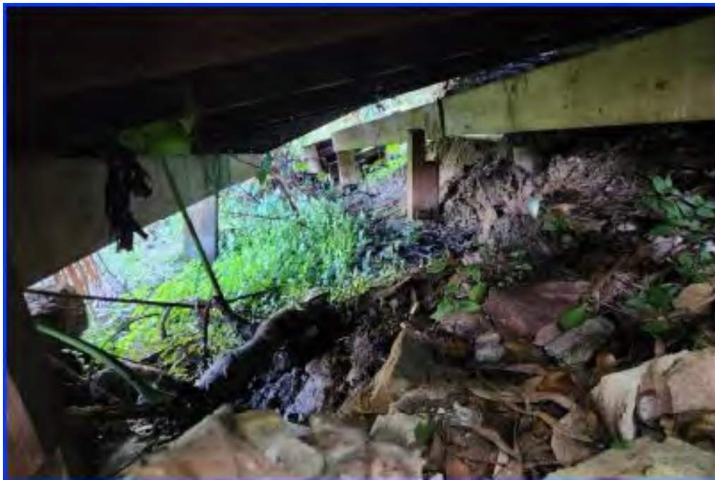
Photo 8-looking south-west under the lower deck showing a possible backscarp.
