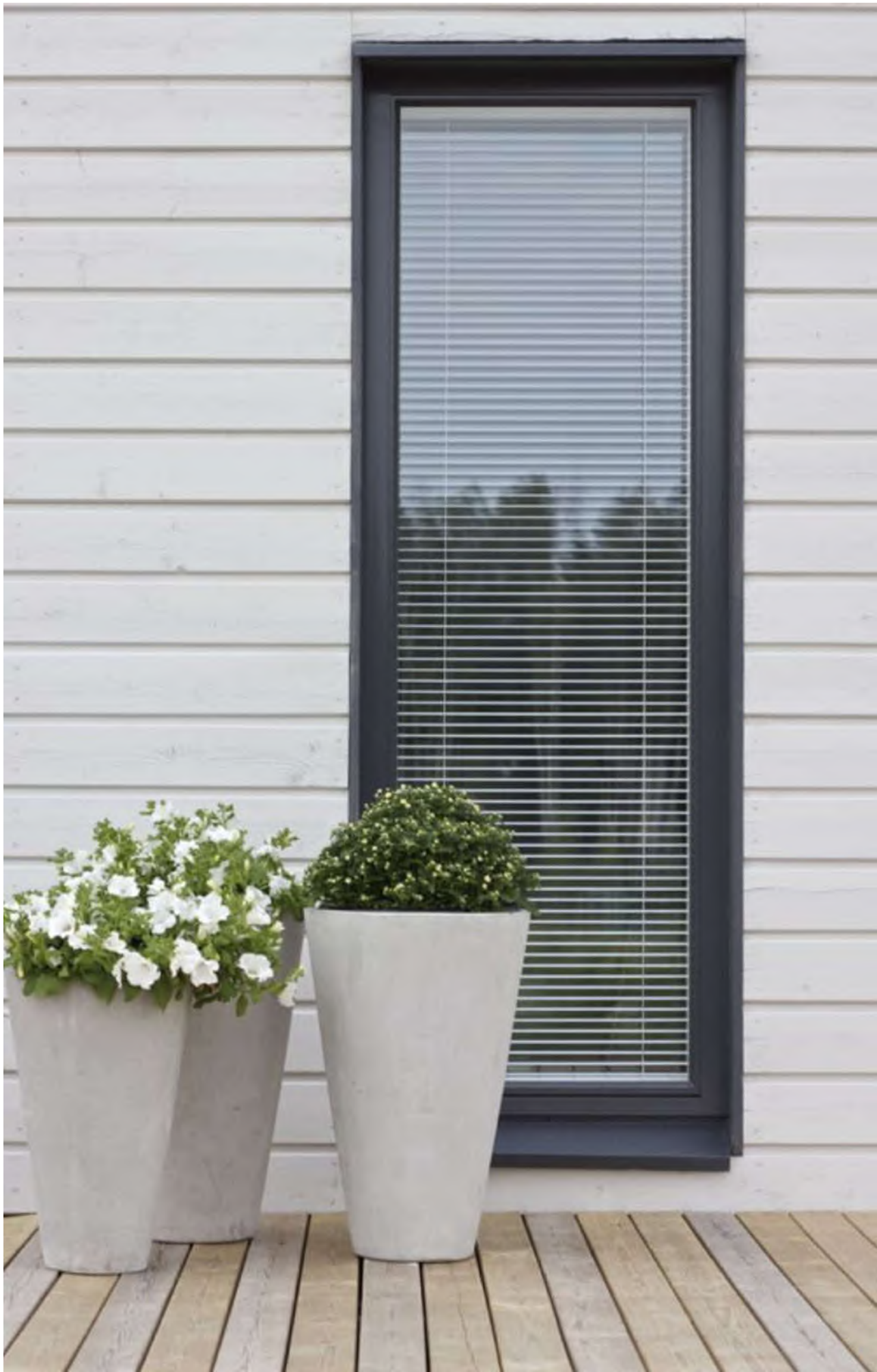
Dark Window Frames, Timber Type Deck
