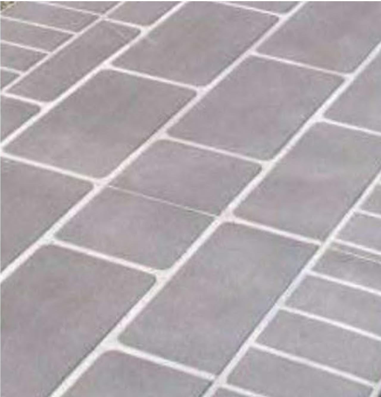
Driveway and Paths - Concrete / Stenciled Concrete Finish
