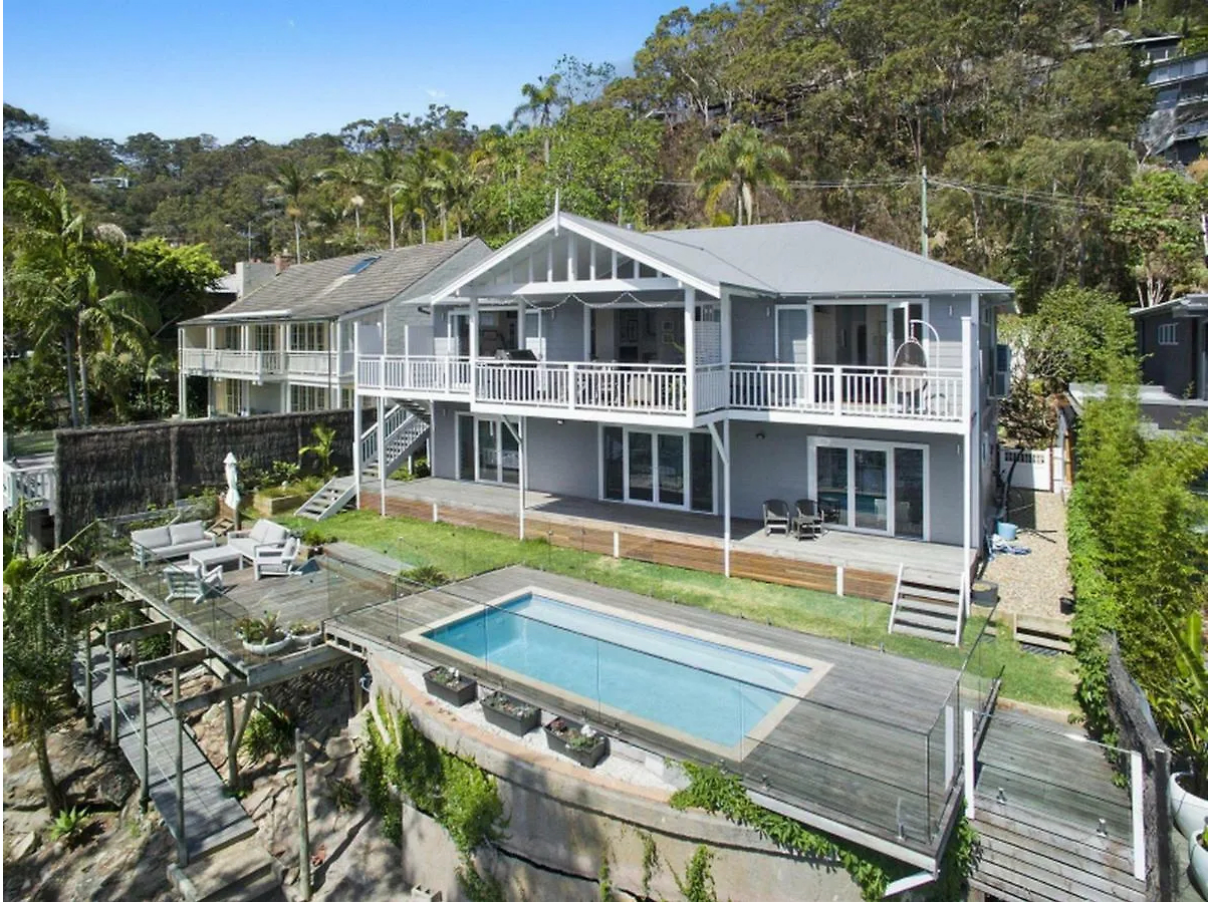
Figure 1: External View of house prior to Landslip Event, March 2022.
