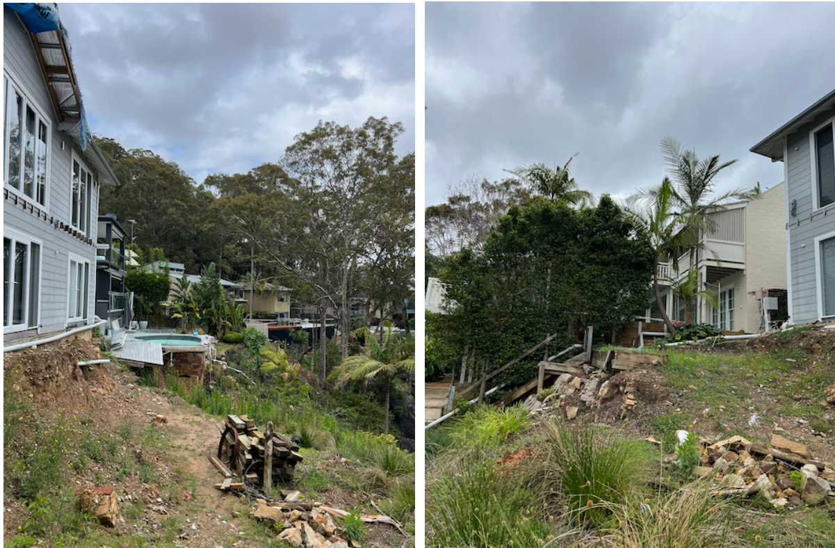
Figure 3 and 4: Current conditions at the site (Foreshore area) December 2023.
