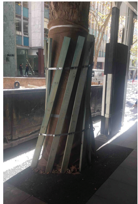
Example of trunk protection installed around a tree
