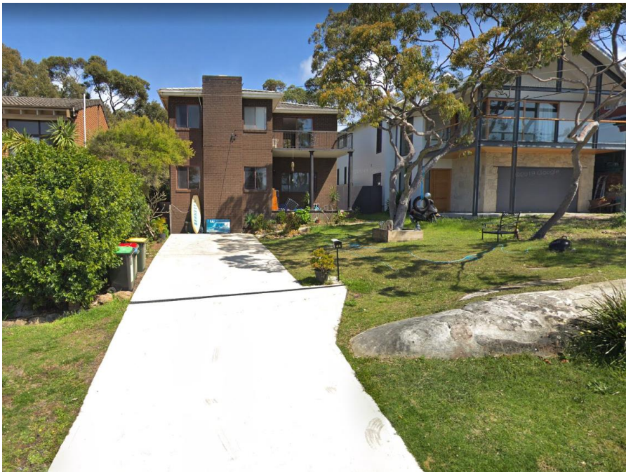
Looking west towards the subject site.
