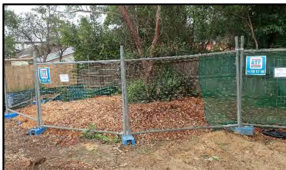
Image: Good tree protection fencing as per AS 4970 – 2009. Image Paxton.
