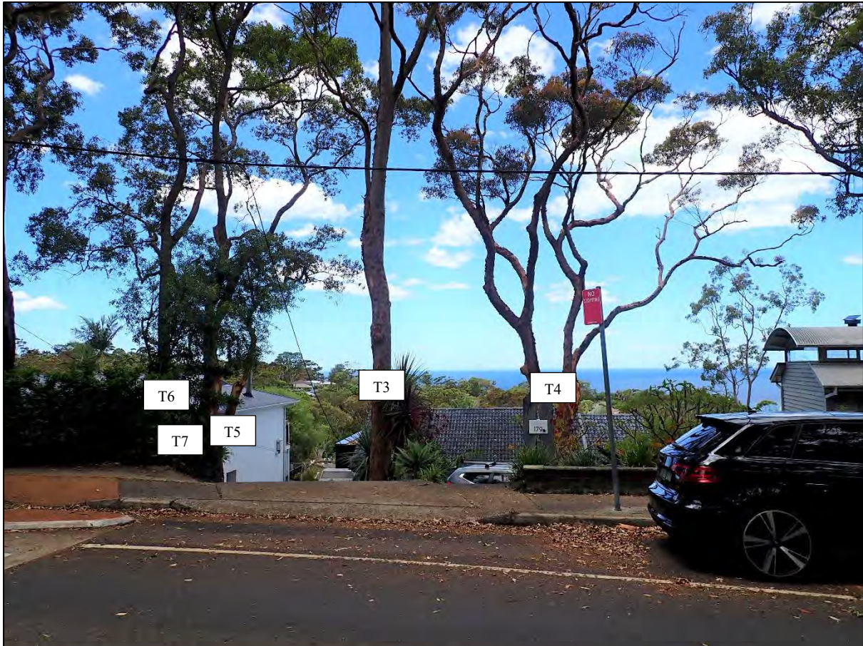
Image 22, Overall view of the site .
