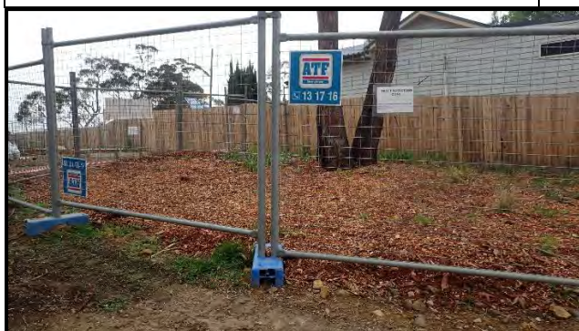
Image: Good tree protection fencing as per AS 4970 – 2009. Image Paxton.
