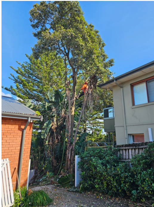
Photo of Tree 6 being removed
