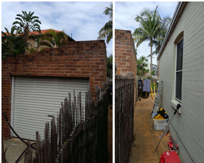
Figure 6 View of the adjacent garage to the east
