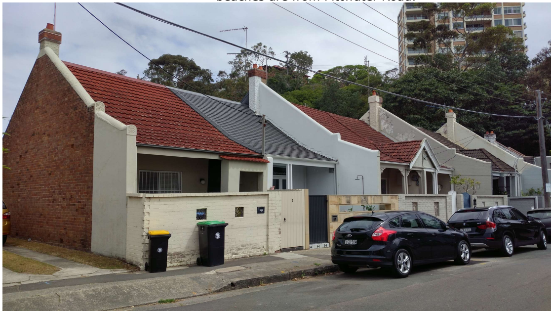
Figure 3 View of the front of the site from Carlton Street.
