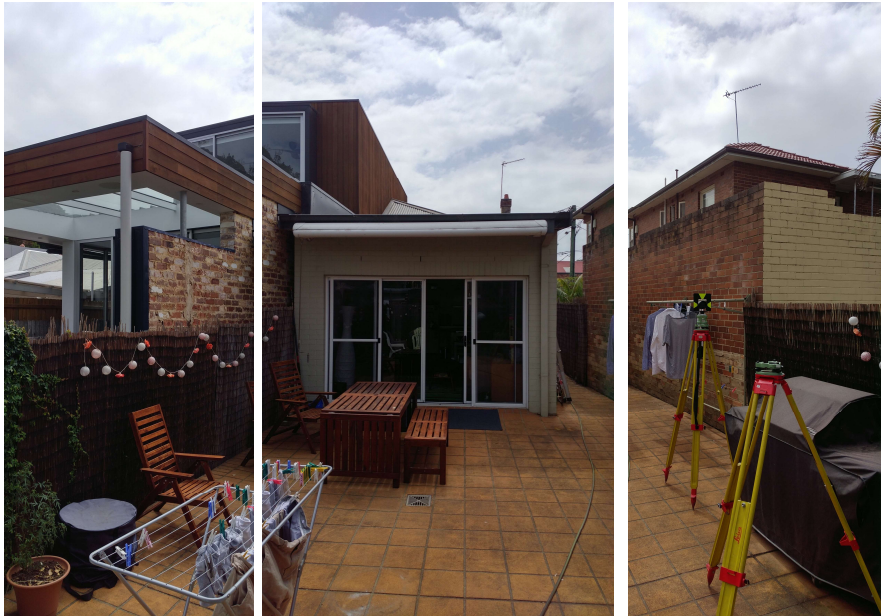
Figure 4 View of the rear court & dwelling
