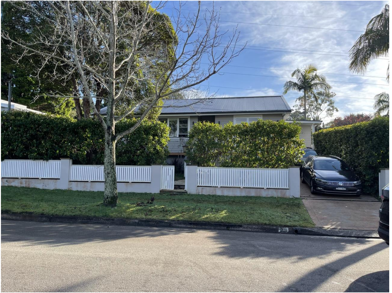
Figure 6. Existing front fence
