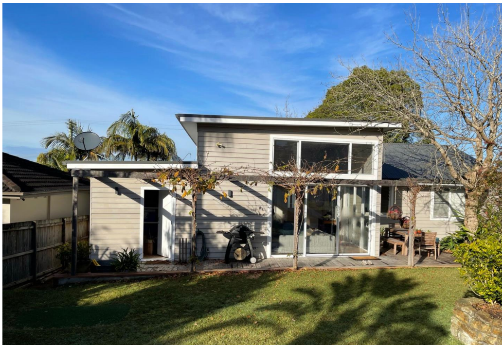
Figure 5. The existing rear of the dwelling, view (looking south)
