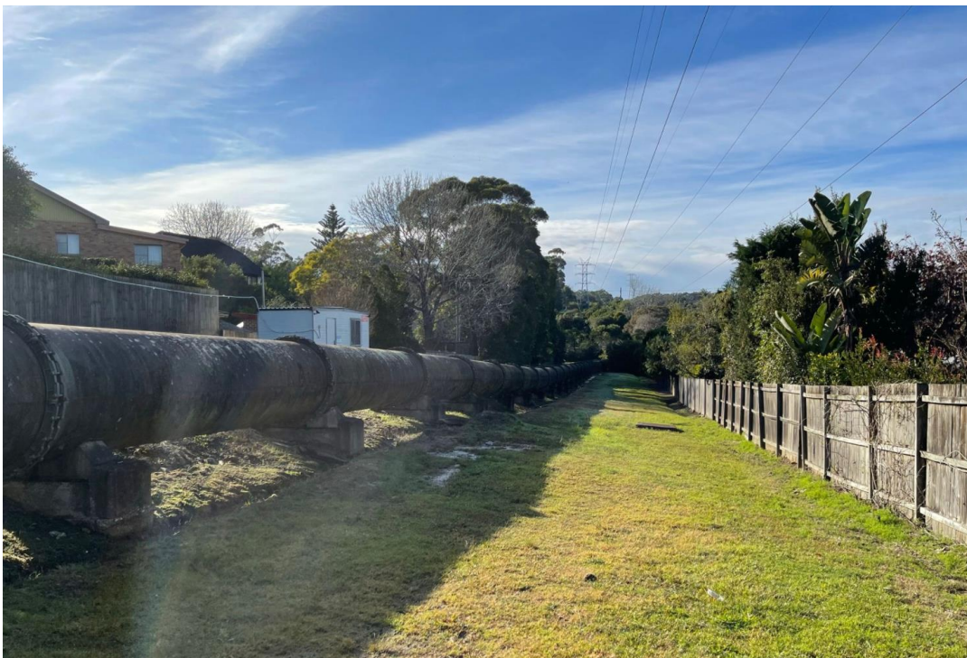
Figure 7. Reserve at the rear of the subject site (looking east)
