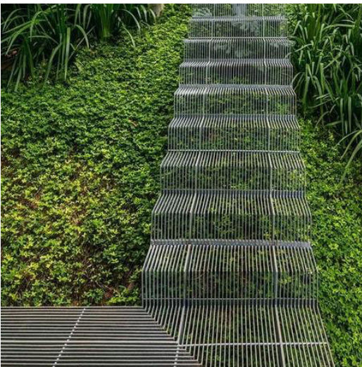
OPEN METAL TO ENTRY PATH
