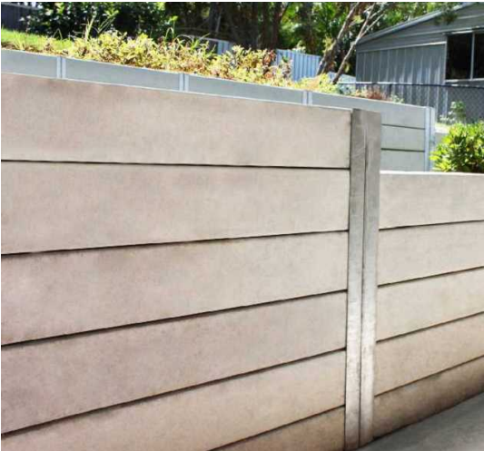
Concrete sleeper retaining wall
