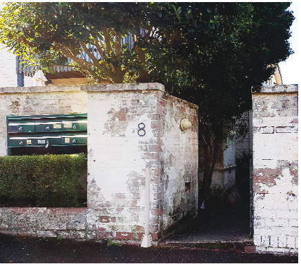
EXISTING ENTRY TO SITE FROM OCEAN ROAD
