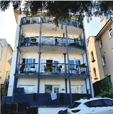
EAST ELEVATION. rear of building
