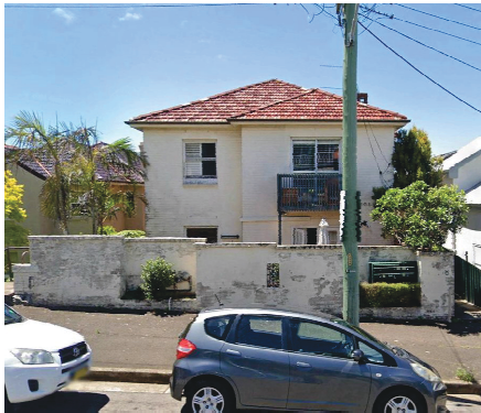
EXISTING VIEW FROM OCEAN ROAD google earth streetview
