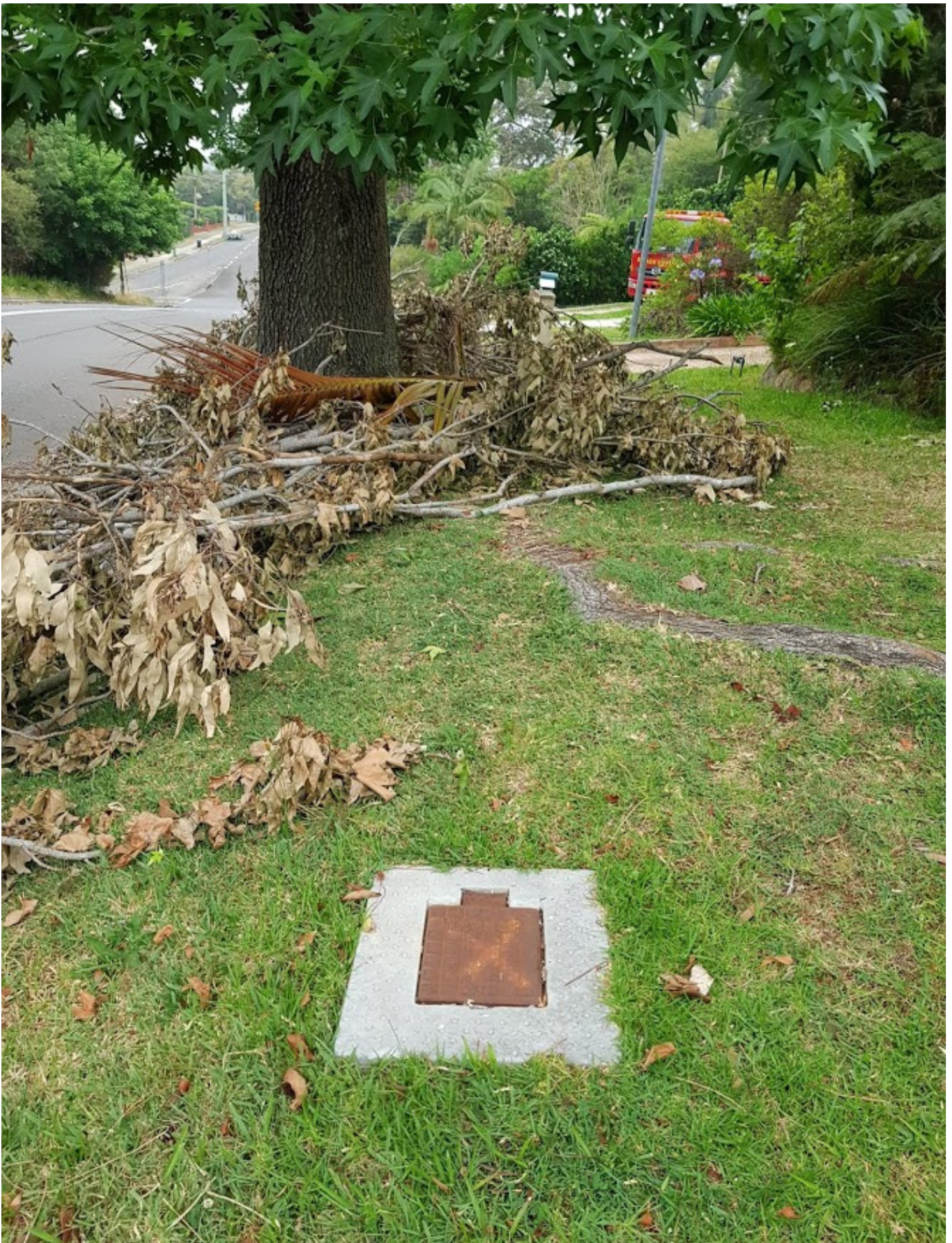
7: Fire hydrant within 20m of the boundary of the site.
