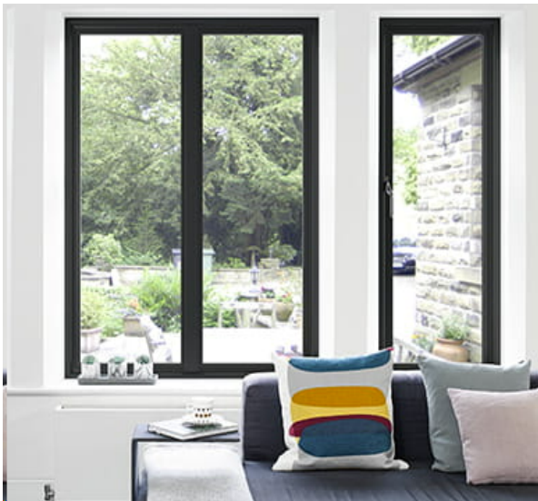
ALUMINIUM WINDOW FRAME POWDERCOAT FINISH 'BLACK' OR SIMILAR TO BE CONFIRMED BY CLIENT.
