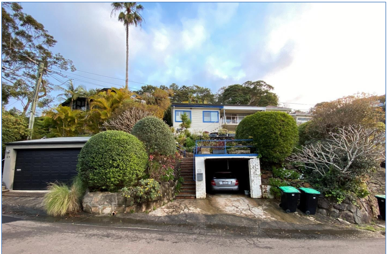
Figure 1. View of subject site of 71 (centre) 67 (left) and 73 (right).
