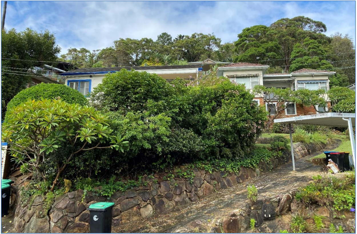
Figure 2. View towards the subject site from the north east, 73 on right, 71 on left obscured by landscape
