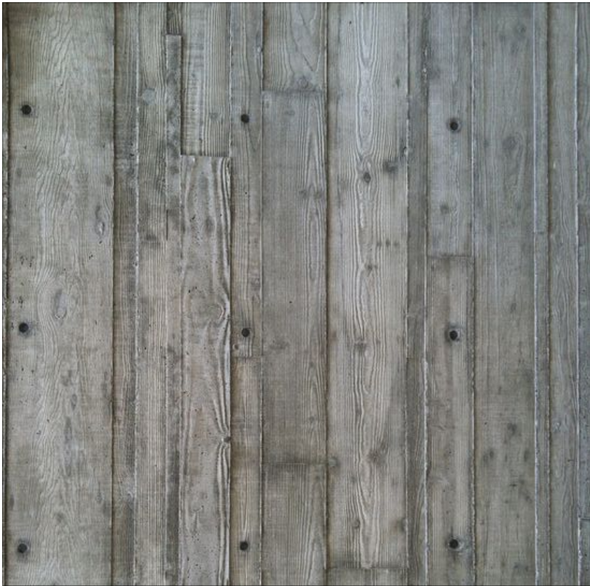
concrete board form
