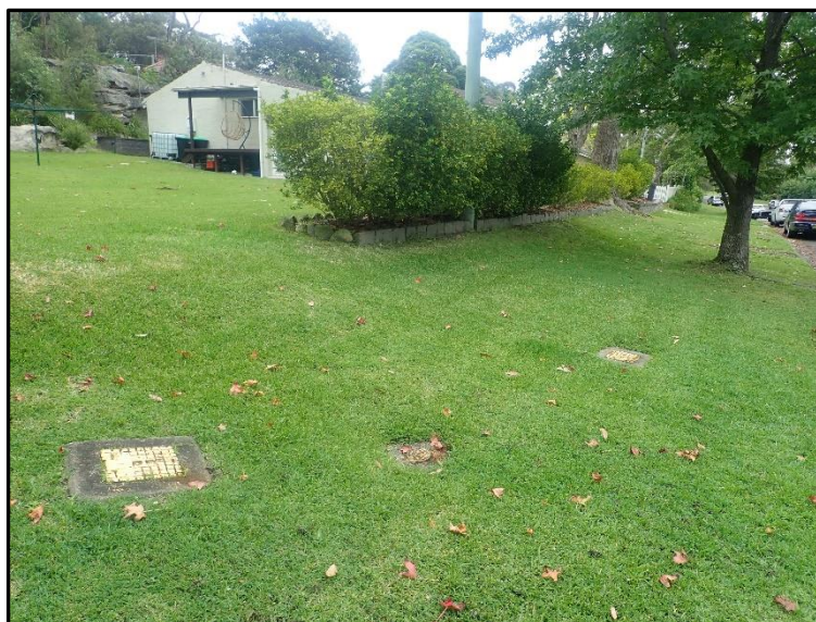
Photograph 05: View west from Coleen Avenue showing existing hydrant location.
