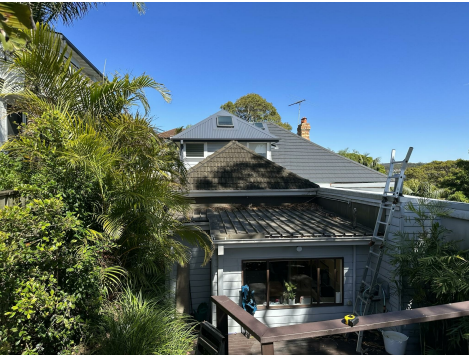
3. VIEW OF PROPOSED AREA OF WORKS
