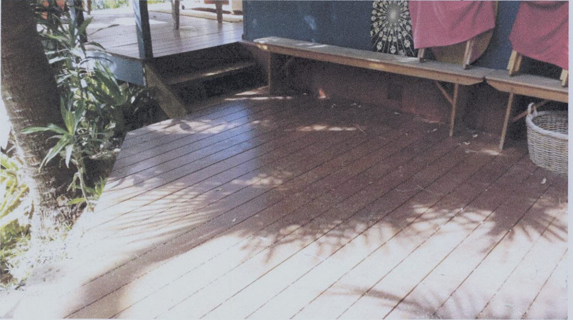
Photo 4 – View of decking boards to west of cottage.
