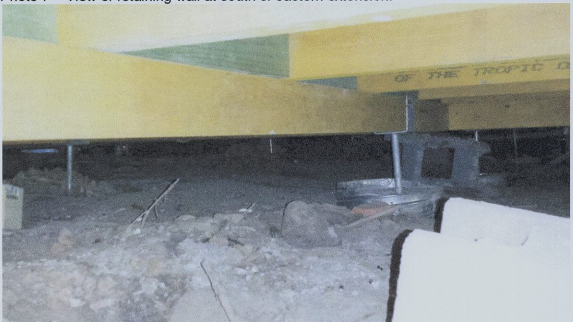
Photo 8 – View of floor framing under eastern extension.
