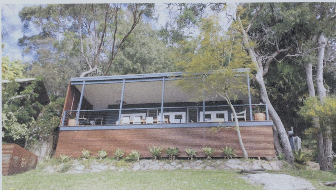
Photo 1 – North elevation of cottage and deck.
