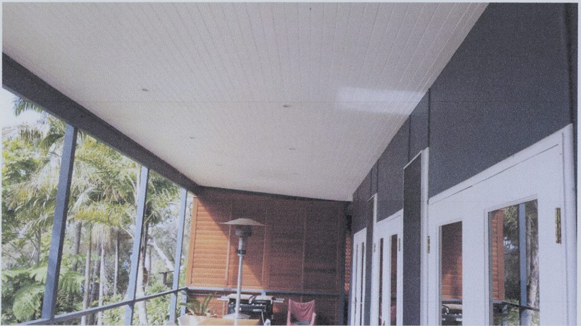
Photo 3 – View of roof framing and posts under northern deck. Note lining boards.
