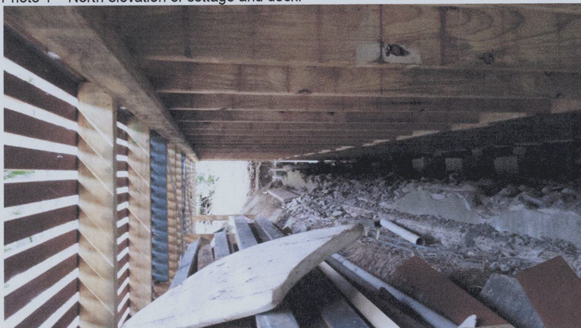
Photo 2 – View of floor framing and posts under northern deck.
