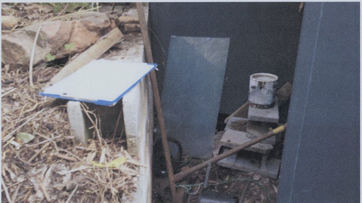
Photo 7 – View of retaining wall at south of eastern extension.
