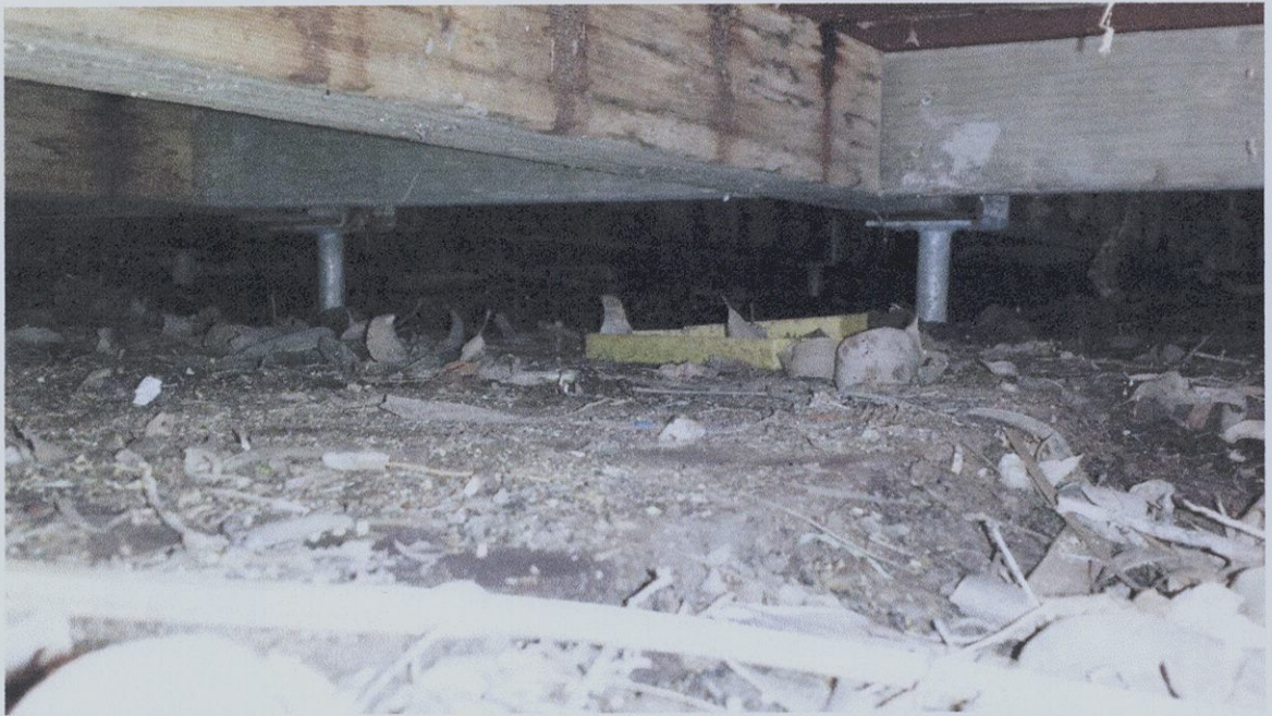
Photo 5 – View of floor framing under decking boards to west of cottage.
