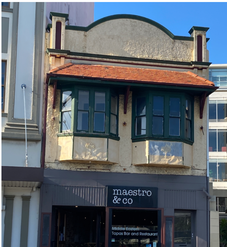
Figure 2: The façade of 50 East Esplanade, Manly.
