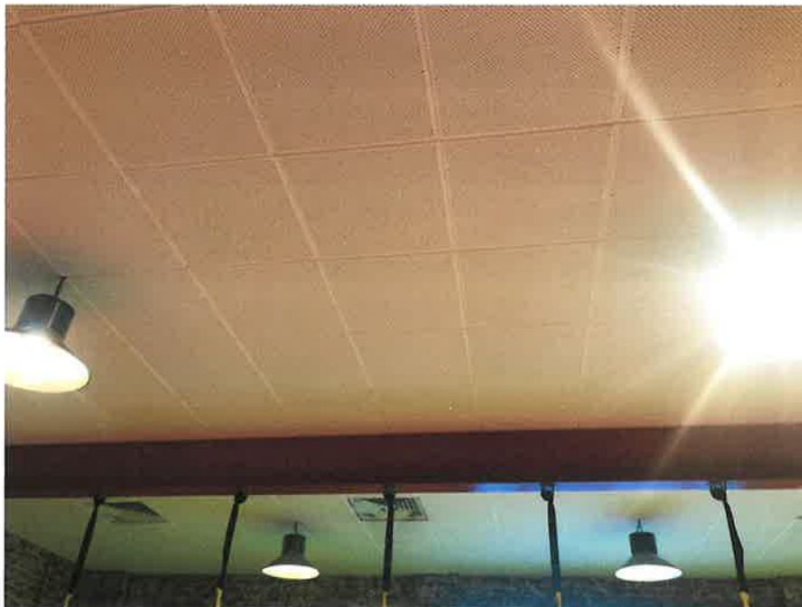
Acoustic Ceiling installed since opening.
