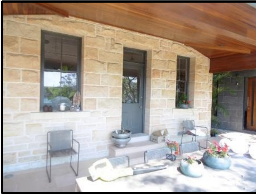
Heritage listed sandstone walled dwelling
