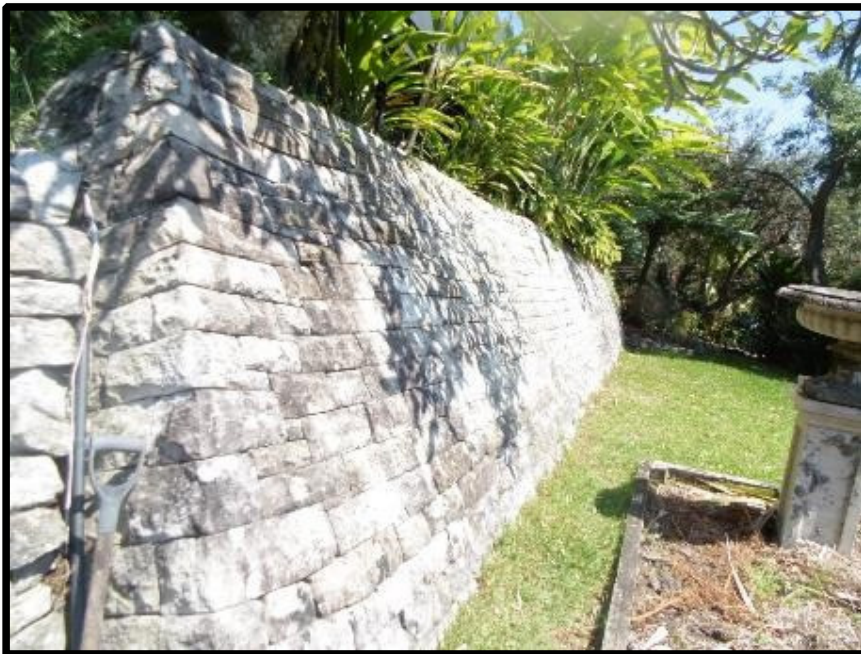
Existing retaining walls to the site
