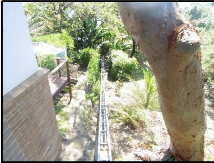
Existing inclinuator to southern side of the allotment
