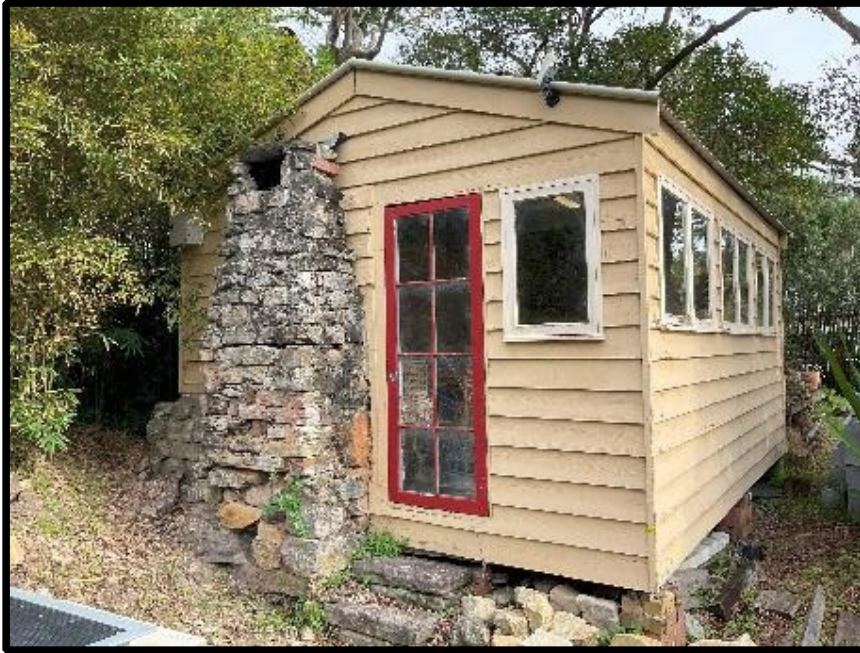
East elevation of boatshed
