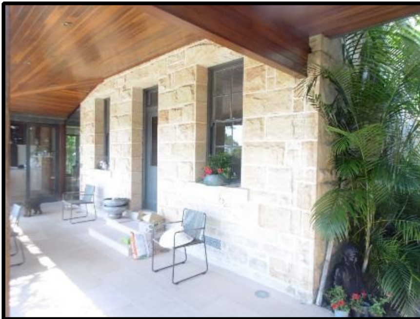
Heritage listed sandstone walled dwelling
