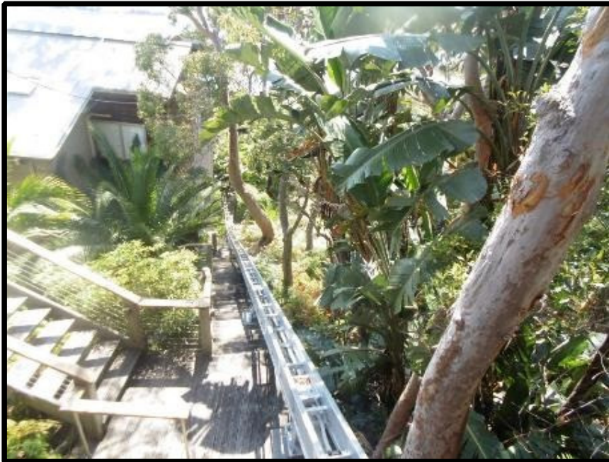
Existing inclinator to southern side of the allotment
