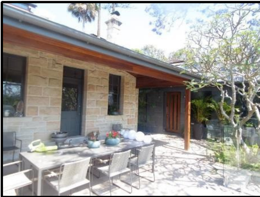
Heritage listed sandstone walled dwelling
