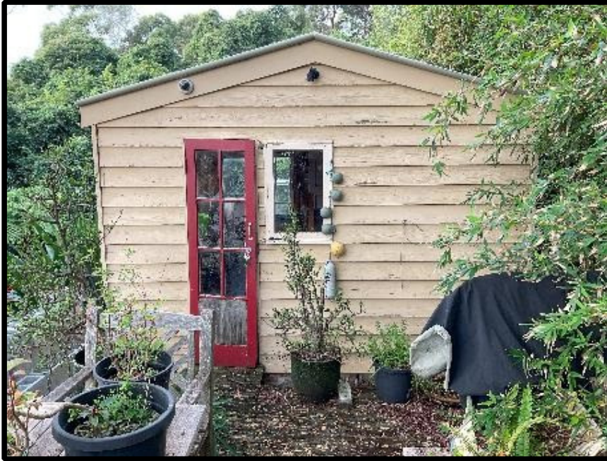
West elevation of boatshed
