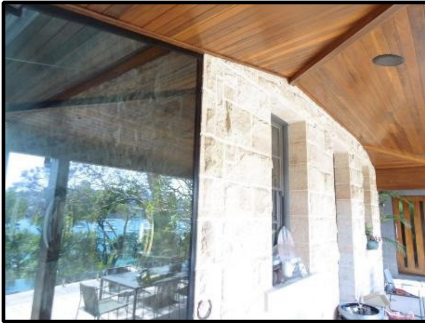
New window to heritage listed sandstone wall
