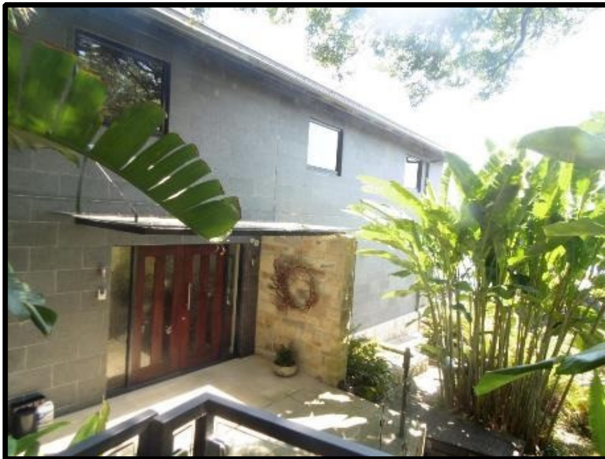
South elevation of whole dwelling
