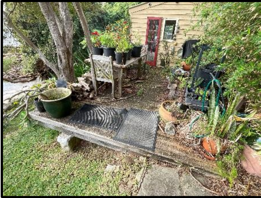
Deck to west elevation of boatshed
