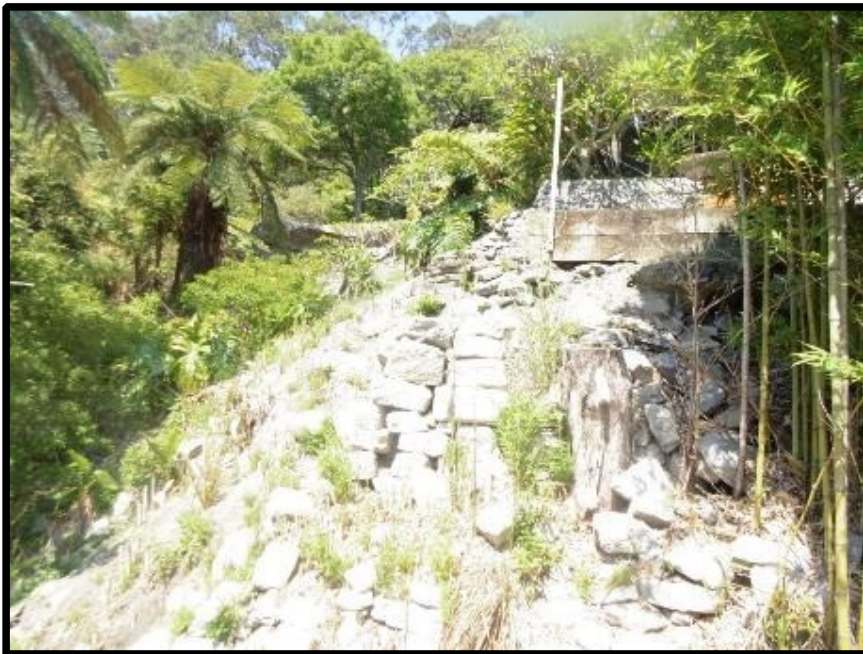
Existing planting and retaining walls to rear garden
