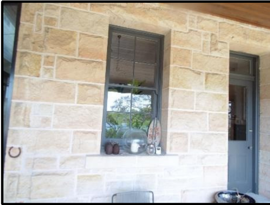
Heritage listed sandstone walled dwelling
