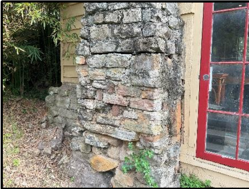
Chimney to elevation of boatshed
