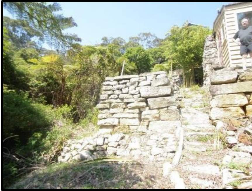
Existing drystone wall
