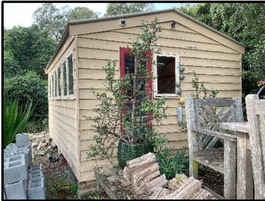
West elevation of boatshed
