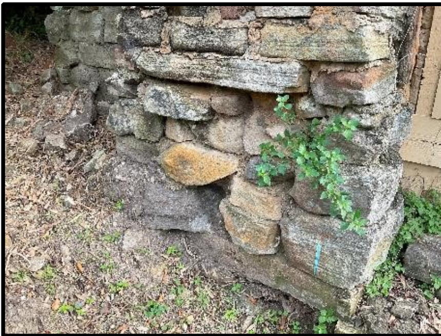
Chimney to elevation of boatshed
