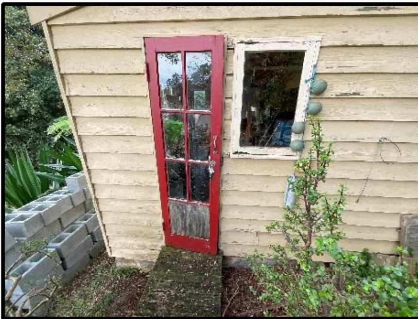
Door to west elevation of boatshed
