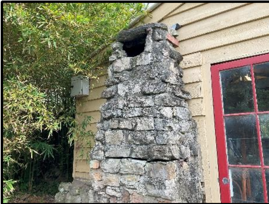
Chimney to elevation of boatshed
