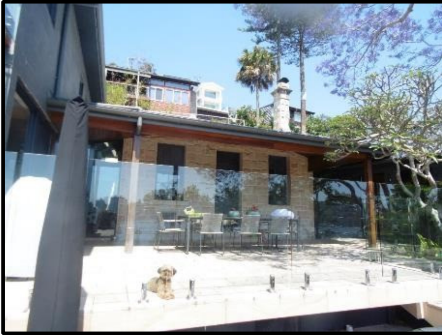
Heritage listed sandstone walled dwelling
