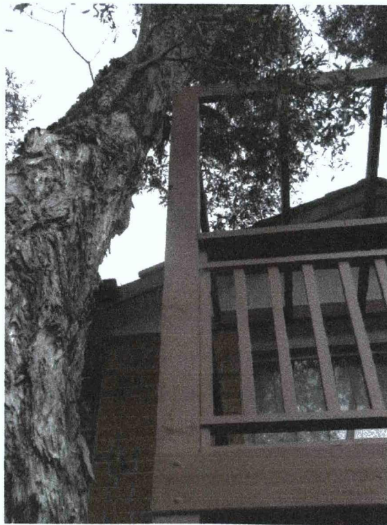
Photograph 2: Illustrating the immediate proximity to the upstairs veranda structure.
