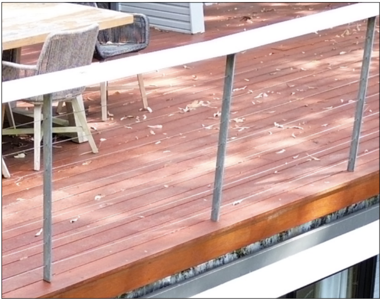
02 - EXTERNAL WIRE HANDRAIL TO MATCH EXISTING
