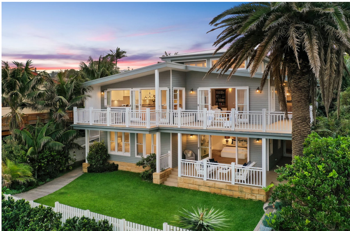
Figure 4. Rear elevation of existing dwelling
